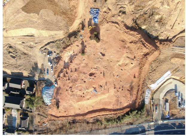
Fig. 2. General view of the excavation site at Area 2~4.
