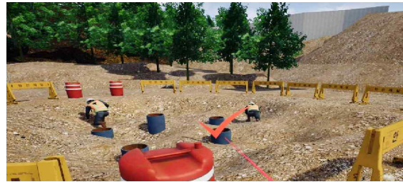
[Fig 5] Road construction Safeline VR content Case
