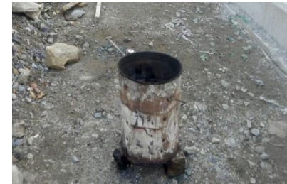
<Fig 14> Temporary Stove Made of Engine Oil Can.
