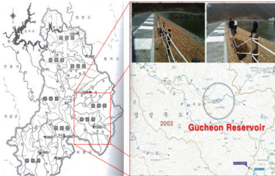
Figure 6. Location of Guchun agricultural reservoir and photos of collapse accident in 2014
