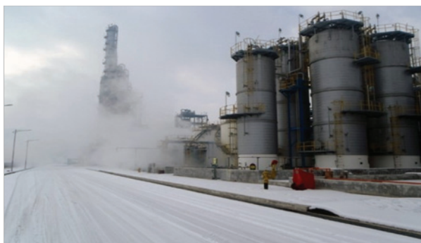
Figure 1. Spill of hydrogen chloride in Kyeongbuk in 2013
