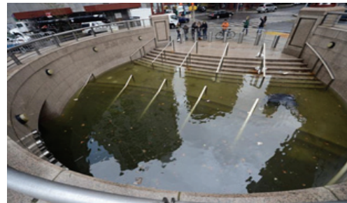
Figure 4. Flooding from Hurricane Sandy
