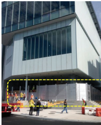
Figure 11. Lobby space protection
