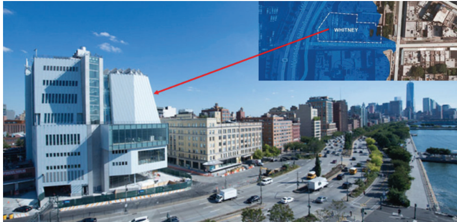
Figure 9. Whitney American Art Museum aerial view with flooded area nearby
