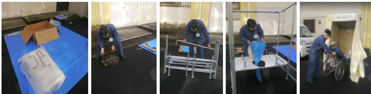
Figure 4. Assembled restroom installation process (Photograph and participation by researcher)
