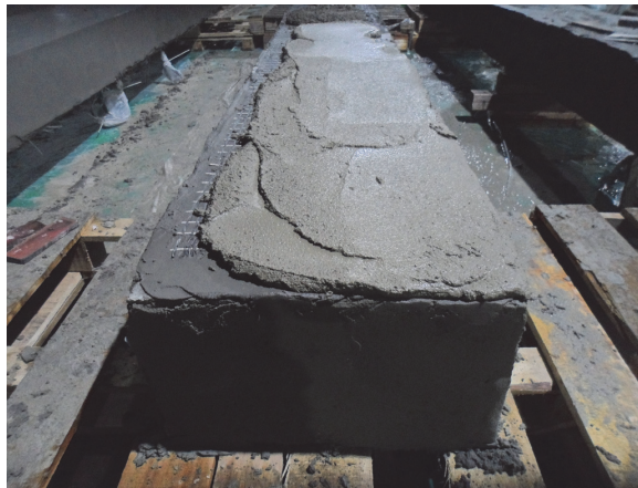
Figure 1. Coated concrete slab beam with polymer cementitious matrix as fire protection
