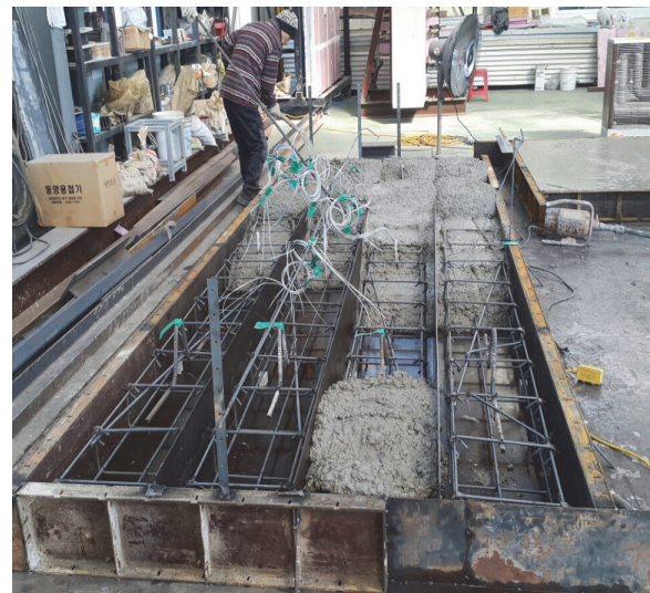
(b) Placing of concrete
