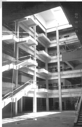
Fig. 12. Chang sha central Hospital
