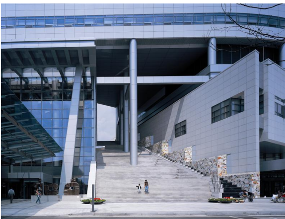
Figure 14. New Yonsei Severance Hospital - Grand Stairway
