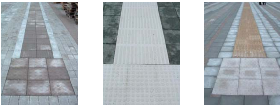
주) Trafikverket - Swedish Transport Administration, 2004
