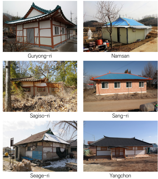
[Fig. 2] Picture of Secondary Station in Dangjin
