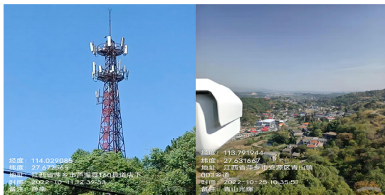
[Fig. 22] The high point monitoring of the communication operator's base station
