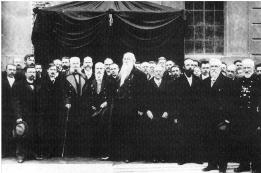
<그림 2 > The laying of the foundation stone for the reading hall designed by Yevgraf Vorotilov. Photograph by Karl Bulla. 1896 출처: http://nlr.ru/eng/nlr/history/5.htm
