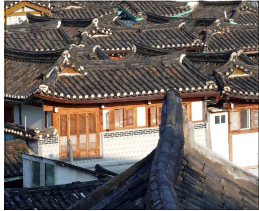
Figure 6 _Hanok in Bukchon, Seoul
