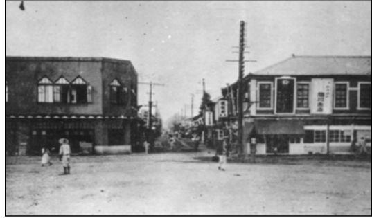
Figure 9 _ Landscape of Suwon Station During the Japanese Colonial Period
