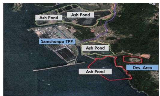
Fig. 5. Application of a side wall using coast shoreline for revetments block
