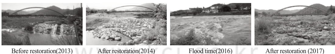
Figure 7. Before and After Site Views of Restoration at FishWay
