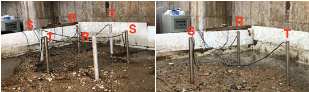
Figure 11. Pilot box experiment for evaluating heat transfer efficiency by hexagonal (left) and triangular (right) arrangement (Type: Pipe, Material: STS 316, Water content: 35%).
