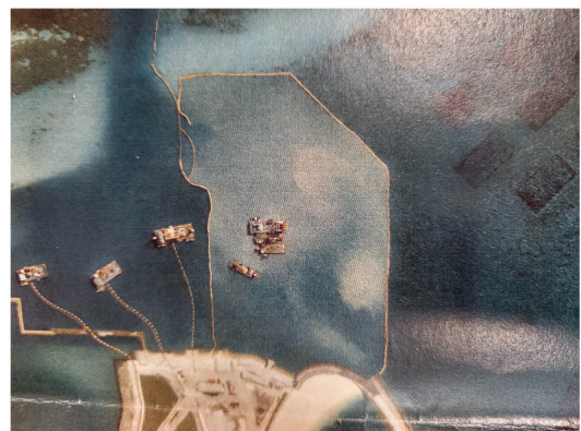
Figure 5. Example of installation of silt curtain during a harbor construction project
