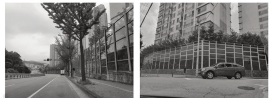
Figure 1. Sound barriers installation section and view in Suwon-si.
