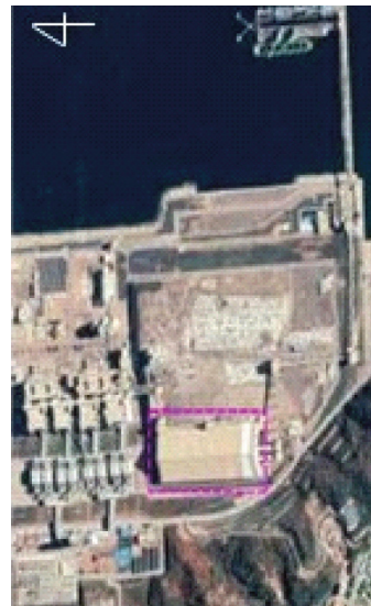
Figure 3. Satellite picture of coal shed in a coal power plant.
