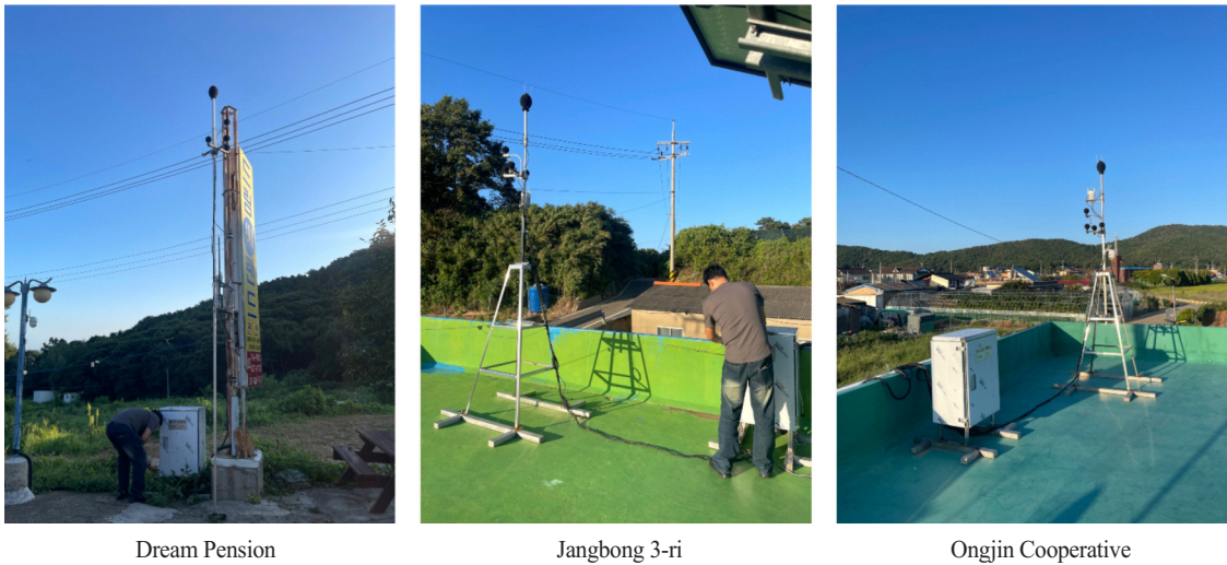
Figure 2. Noise Monitoring Installation Sites.
